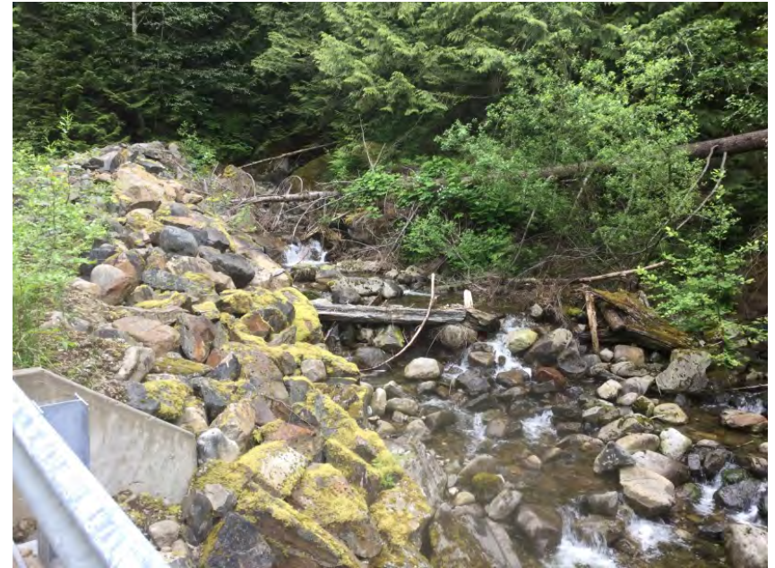
Looking upstream from deck
