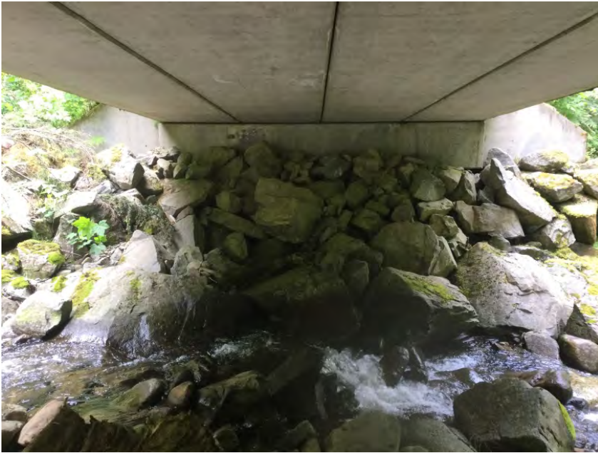
Left Bank Abutment when facing downstream
