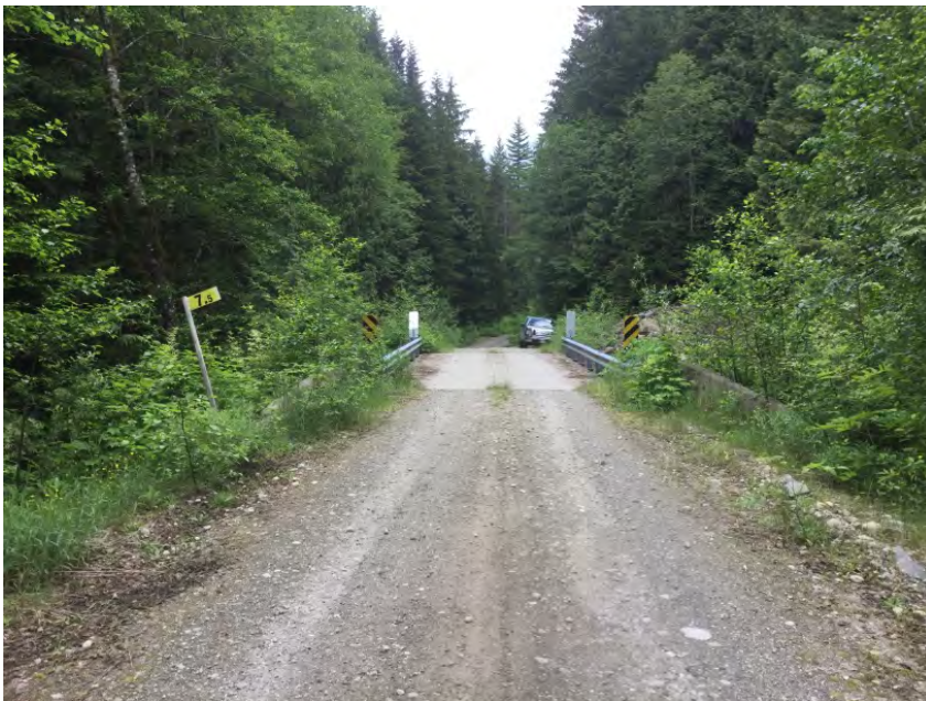
Approach from Left Bank when facing downstream
