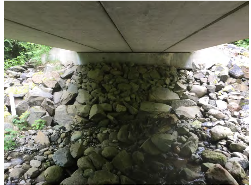
Right Bank Abutment when facing downstream
